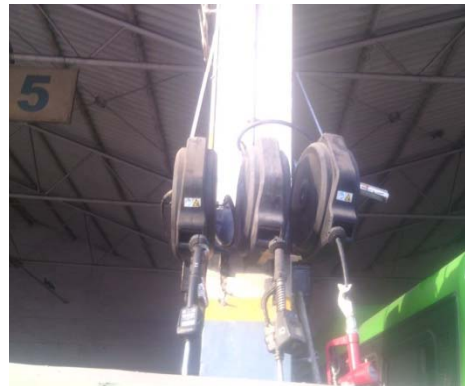
DTC Depot, Subhash Place
