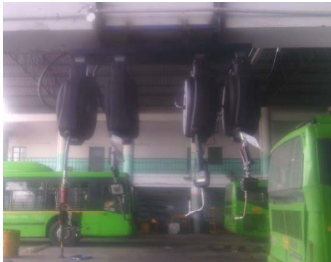
DTC Depot, Dwarka
